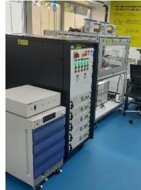
High Voltage lab
