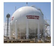
Cooled to ~ (-) 253°C and stored in insulated tanks
