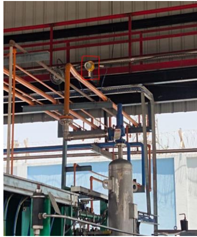
Gas Detector – Compressor B
