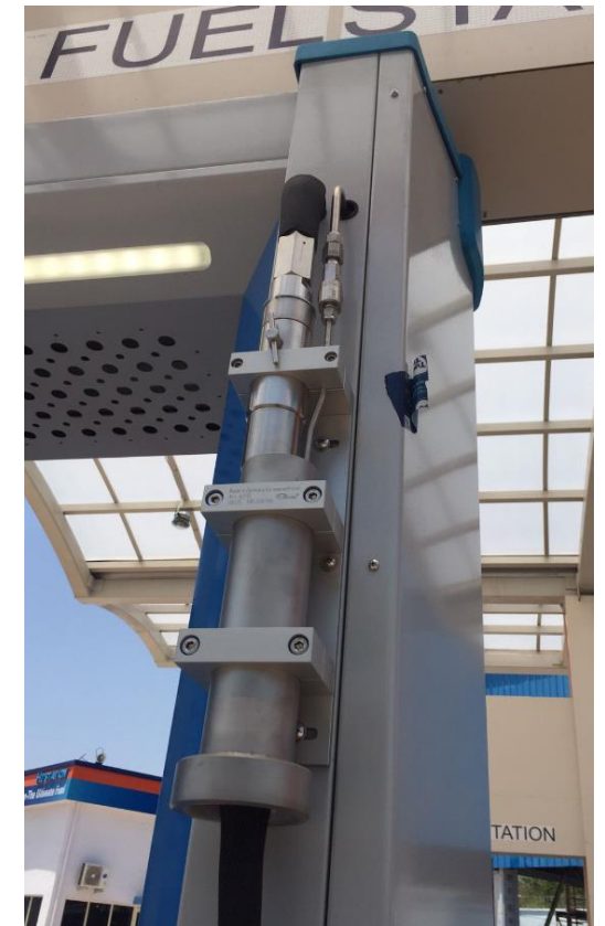
Dispenser-Hose Breakaway Coupling
