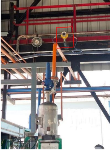
Gas Detector – Compressor A
