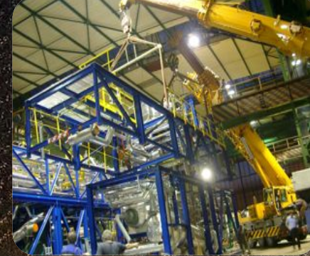
ModuLite™ Shop assembly
