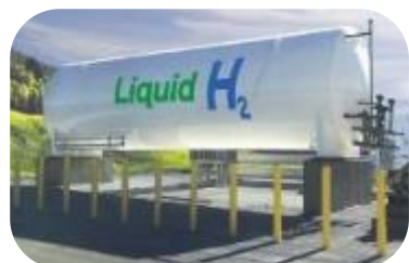
STORAGE TANKS 10 TO 80M 3
